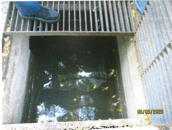
Effluent To Public Pipe
