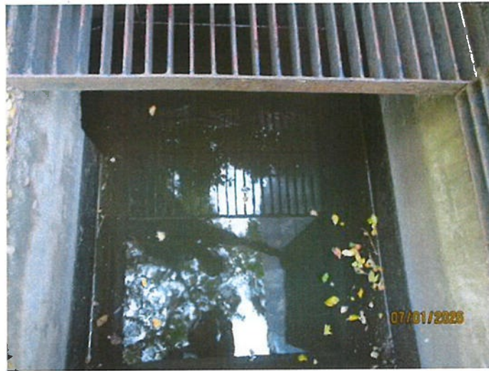
Effluent To Public Pipe
