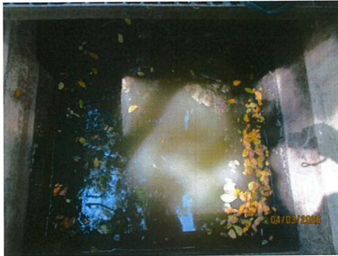
Effluent To Public Pipe
