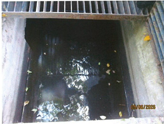
Effluent To Public Pipe
