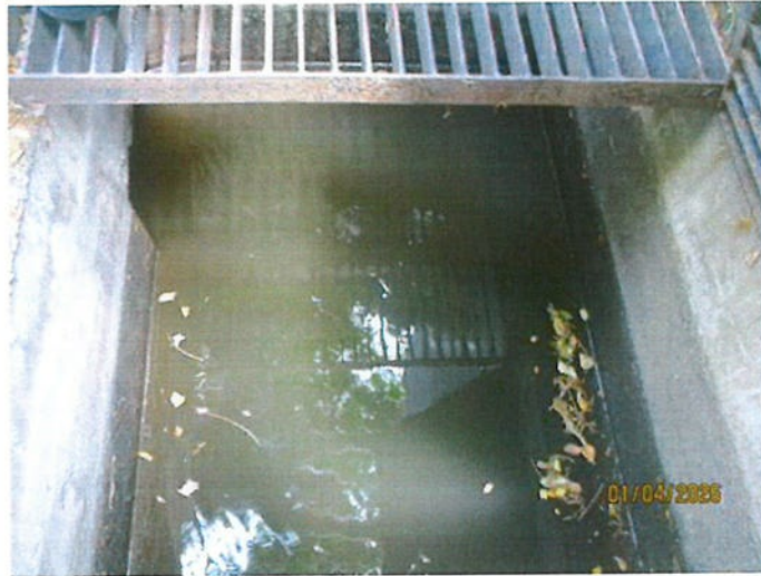
Effluent To Public Pipe
