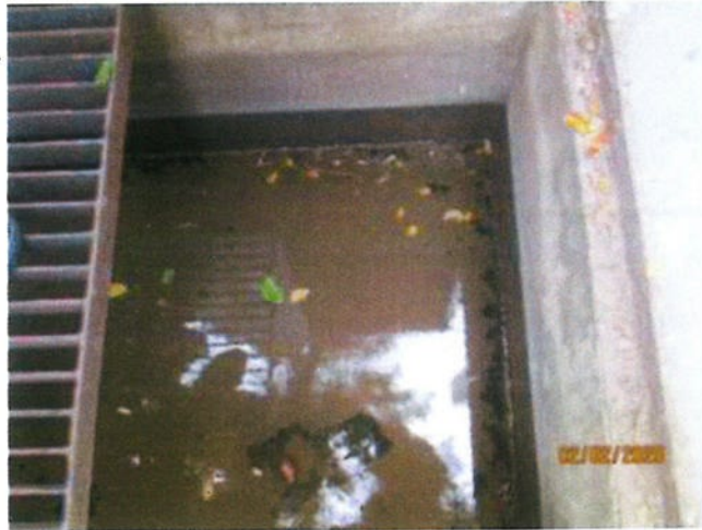
Effluent To Public Pipe
